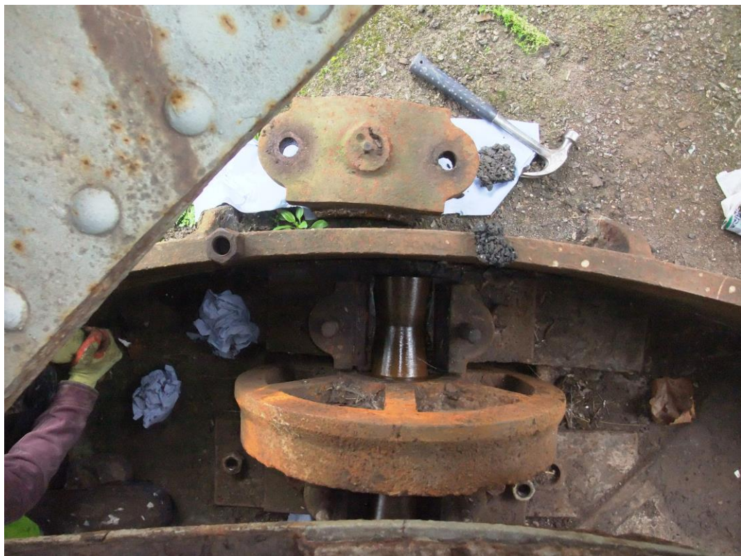
Plate 24 – NE Wheel – Outer bearing
