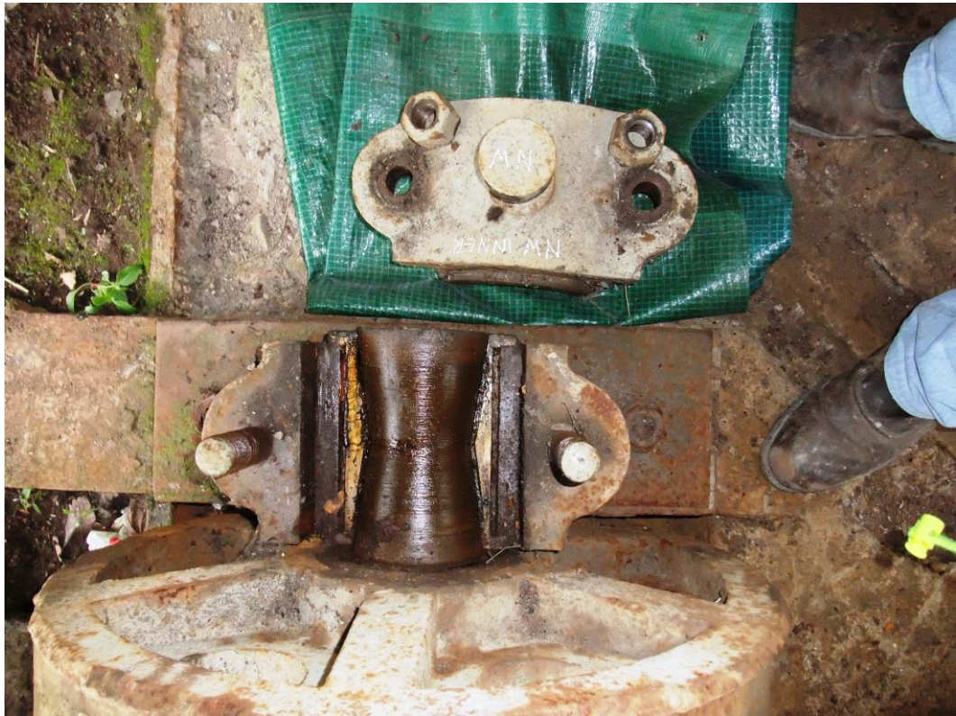
Plate 15 – NW Wheel – Inner bearing
