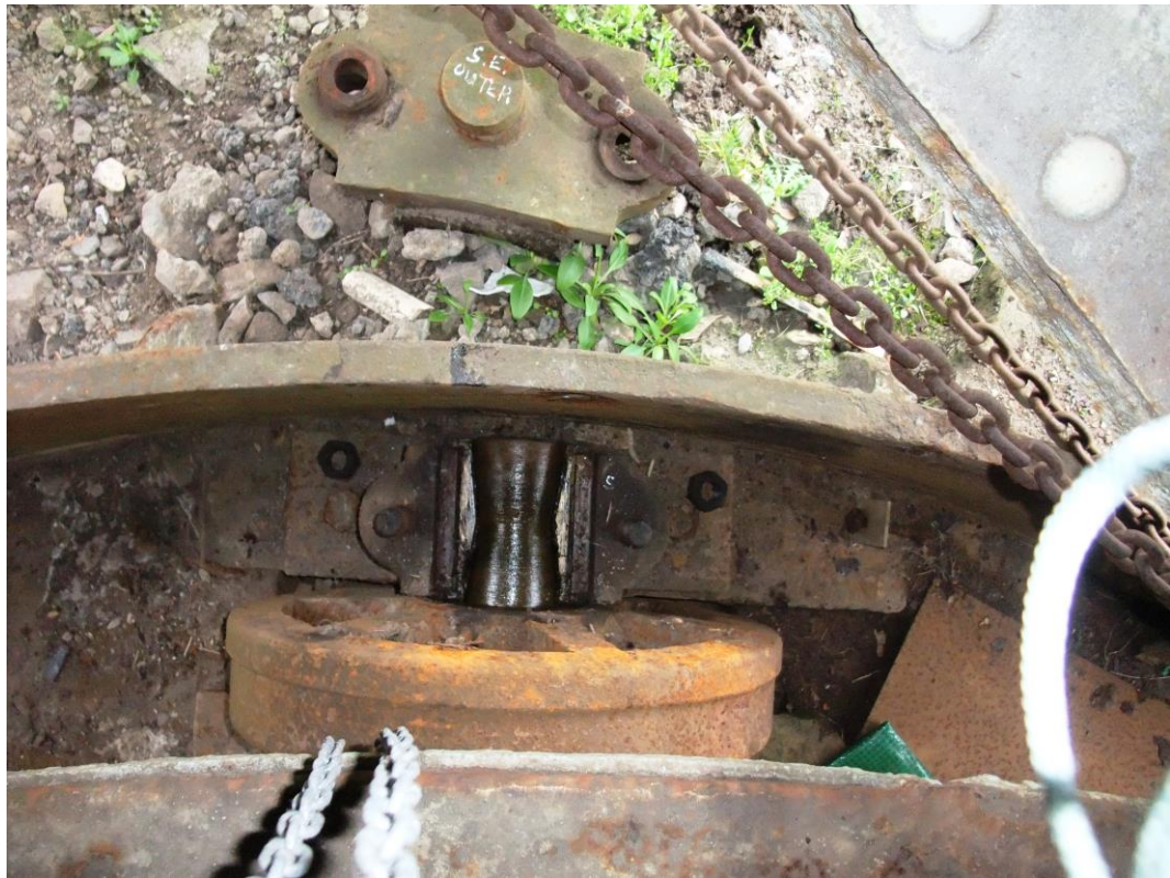
Plate 5 – SE Wheel – Outer bearing
