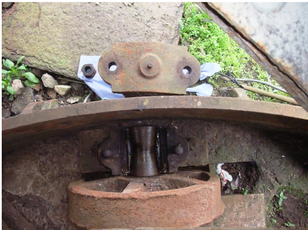
Plate 18 – NW Wheel – Outer bearing
